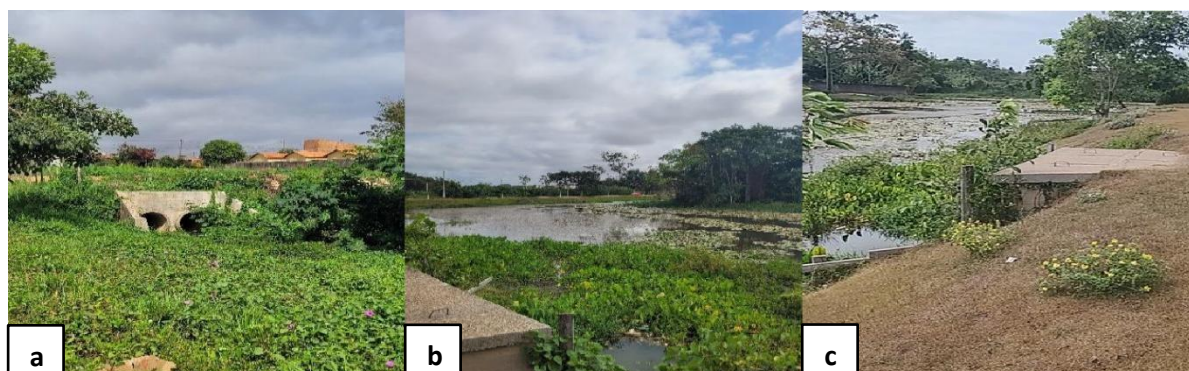
Figure 6. a) culvert through which part of the effluent flows into the Paragominas stream, right bank, direction W → E; b) left bank culvert, direction M → J, in lateral view; c) the same culvert in lateral-frontal view.
