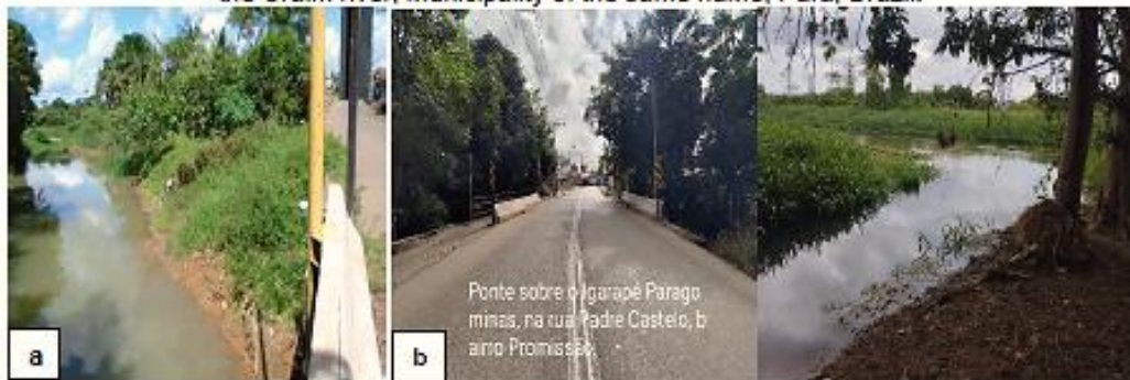
Figure 10. a) Displacement of the water flow from Green Lake to the Padre Carvalho street bridge; b) bridge under which the water flow moves; c) outflow of the Paragominas creek into the Uraim river, municipality of the same name, Pará, Brazil.
